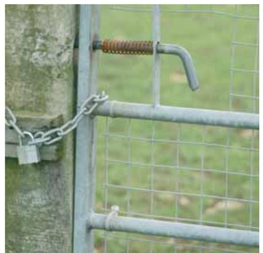
cause injury. Gates should open easily, but steadily, being fixed in such a manner as to give complete control to the operator without risk of either slamming against a horse or swinging beyond the reach of the handler.
